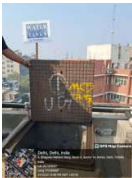
UG TERRACE WATER TANK 2
