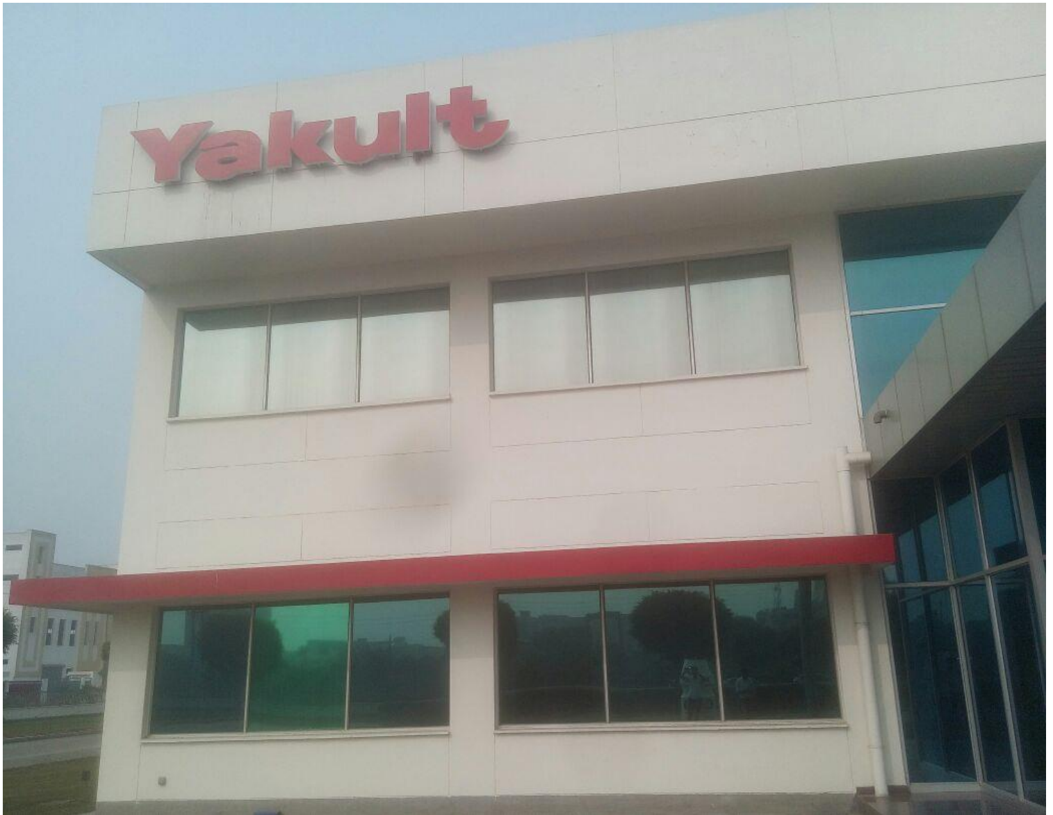
Yakult Danone India Pvt. Ltd. Plant, Rai Industrial Area, Sonapat, Haryana.
